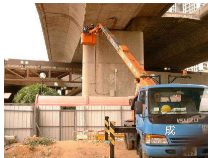
Installation of prism on the bypass
