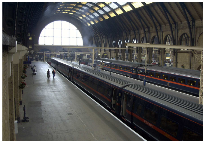
Above : Within the train shed three "CYCLOPS" monitor the internal facades, spine wall and the track sleepers.
