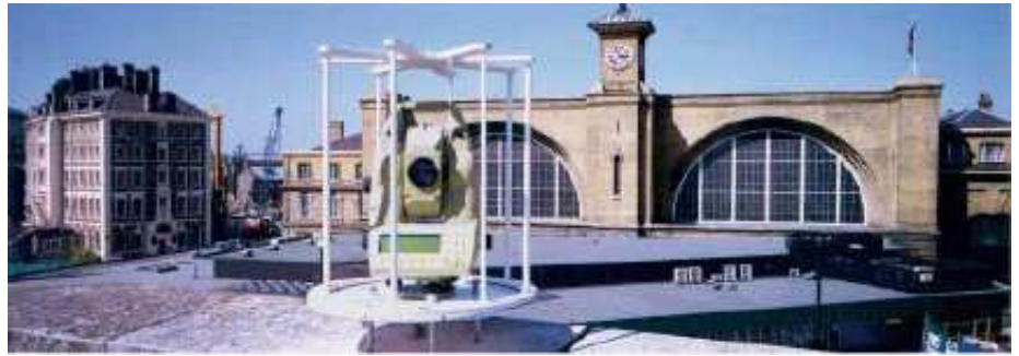
Above : A "CYCLOPS" monitors the southern façade of Kings Cross and the Great Northern Hotel
