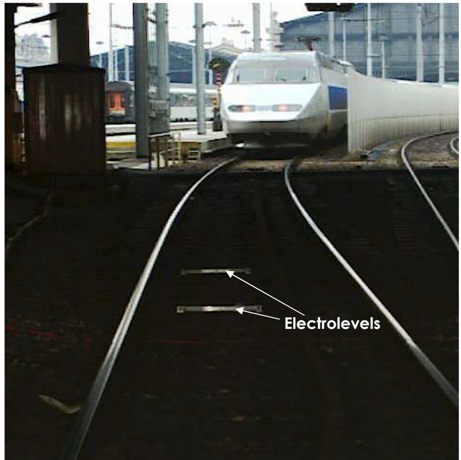
Gare du Nord Terminus: Electrolevels on TGV tracks
