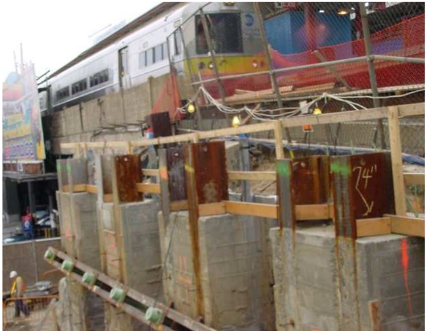
Jamaica station during the extension works
