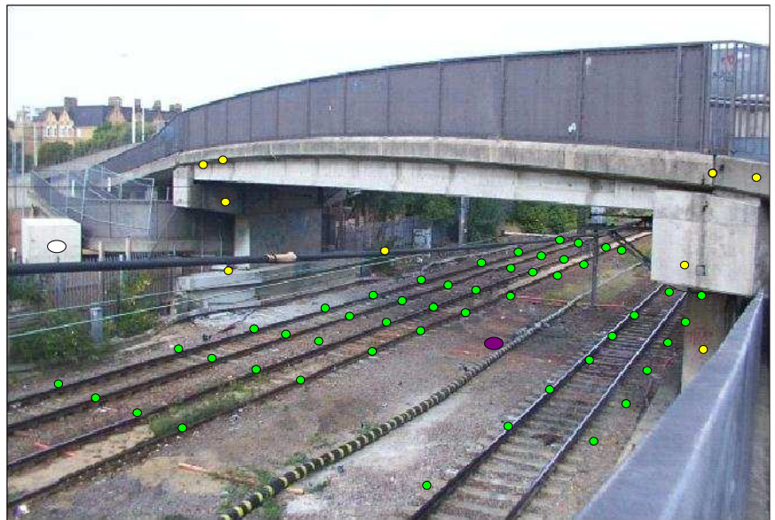
Above: The view from Theodolite B to the monitoring targets. Monitoring targets: Yellow for bridge monitoring, Green for track monitoring, Purple for rod extensometer
