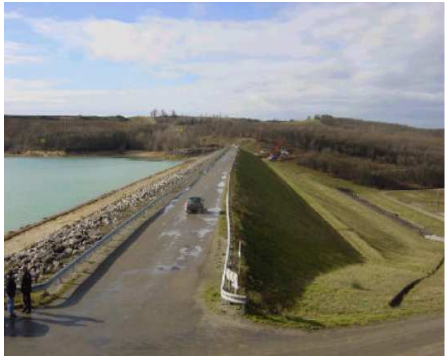
The Ganguise dam from the right bank before the extension works.
