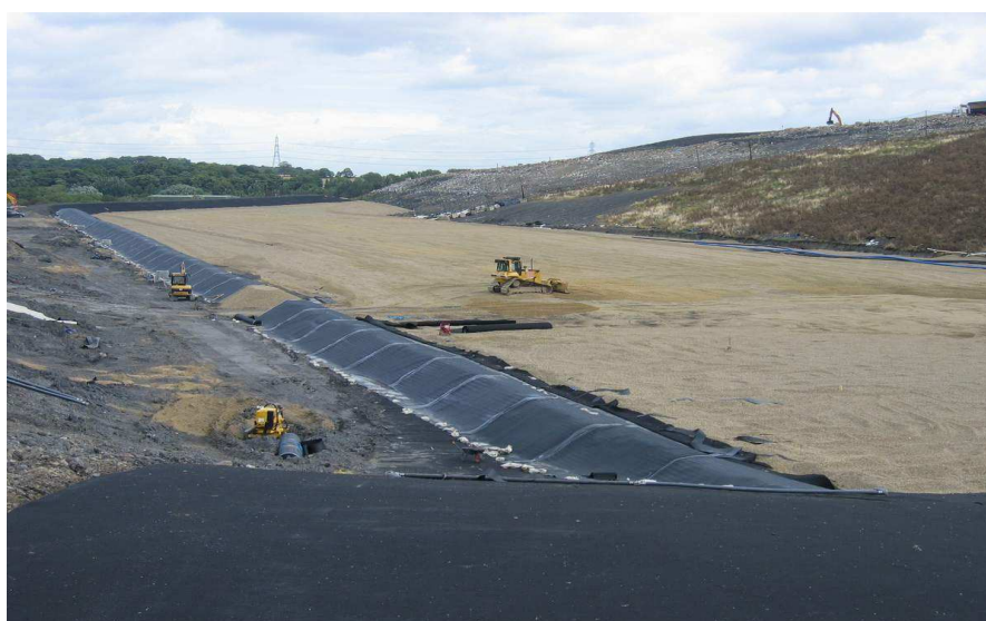
Top left: Installation of settlement cells within foundation trench.
