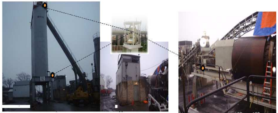
Monitoring of sensitive structures during grouting works
