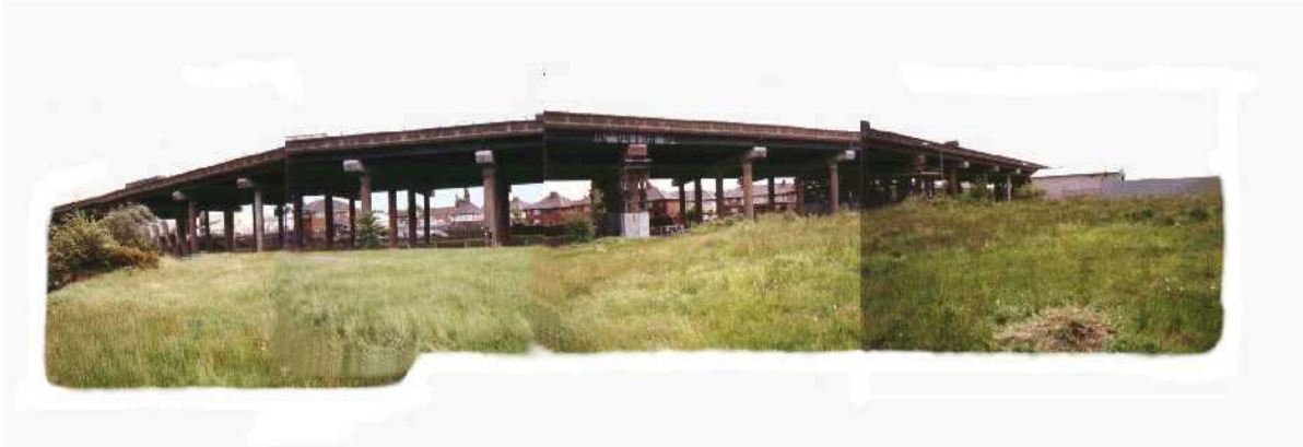
M5 motorway viaduct (Oldbury)
