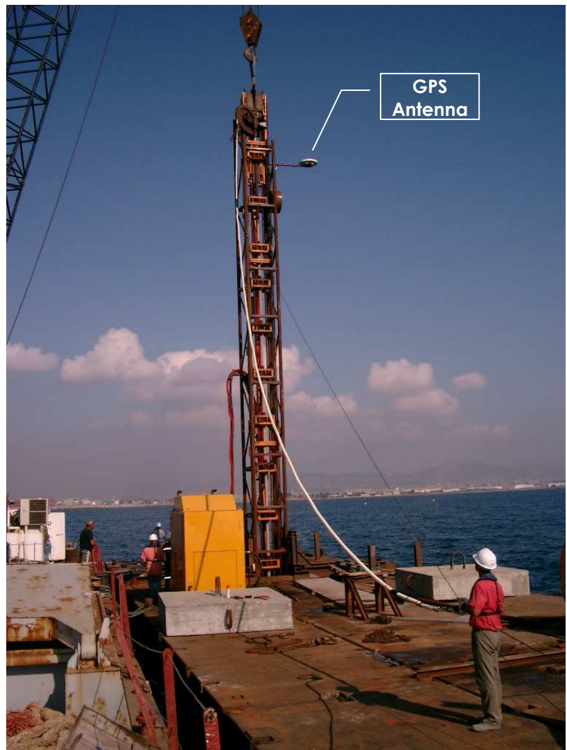
Positioning of the instruments by barge mounted drilling rigs
