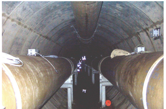
BELOW: view within the tunnel showing geophone arrays
