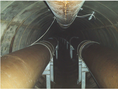
Above (From left to right): View down the tunnel showing the location of one of the CCTV LED cameras. Geophones mounted on the pre-cast concrete lining and the GRP pipes. High precision crack gauge (accurate to 0.1mm) installed over one of the GRP pipe joints.
