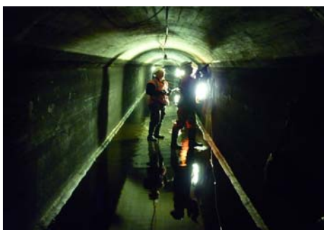
Installing within the conduit during the outage.
