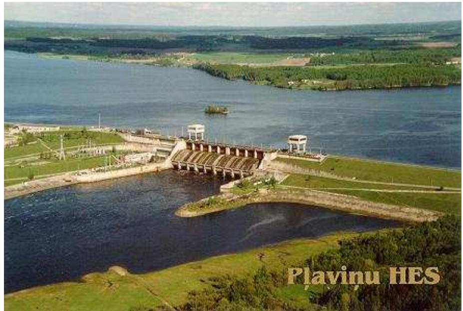
Plavinas Dam (70 m high) The main power station in Republic of Latvia
