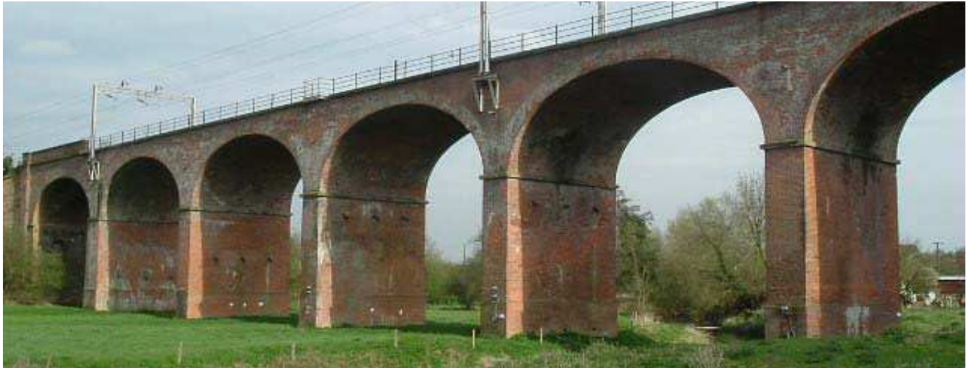
Above: View of the Lexdon Viaduct equipped with accelerometers
